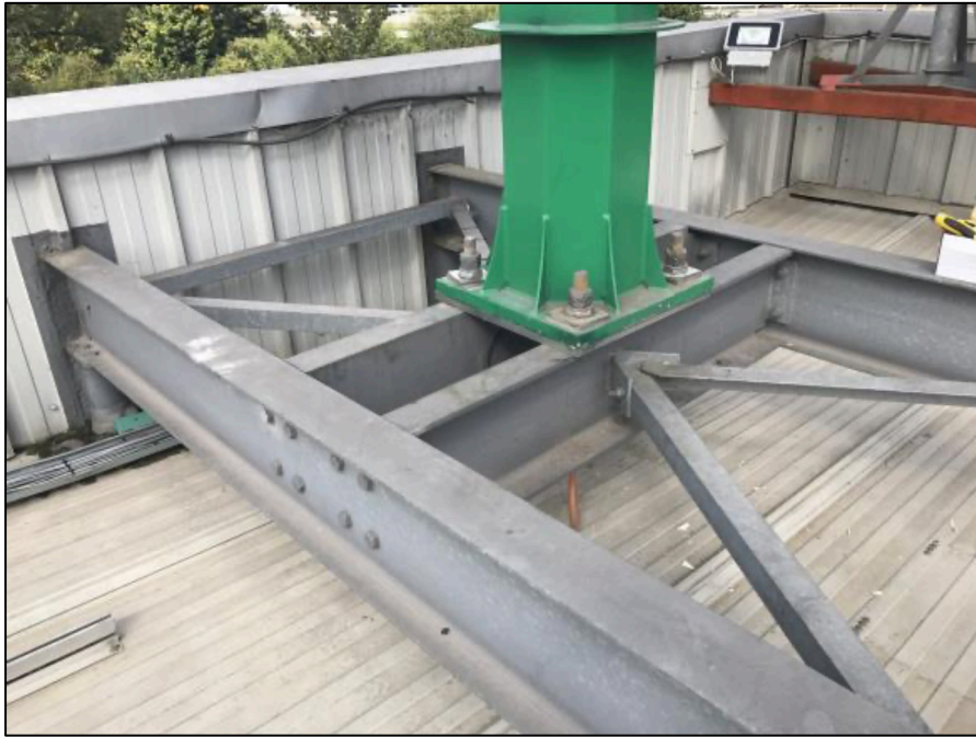
Figure 23: Structure supporting the tower of the Qr6 VAWT [24]
